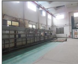
Photo of the inside of the main production hall phosphating line.JPG
