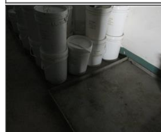
Photo of non-conformity NC-secondary container is insufficient.JPG
