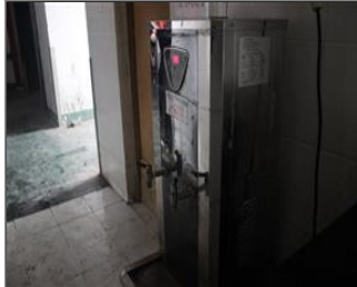
Photo of the inside of the main production hall Drinkable water.JPG
