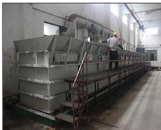
Photo of the inside of the main production hall Phosphorization.JPG
